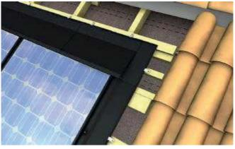
6 Place the precompressed seal on the flashings around the area on the lateral and upper parts.
