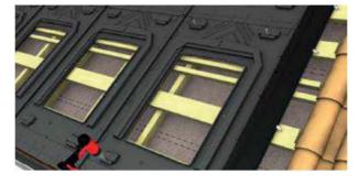
Then, pre-drill the fixing points of the clamps.
