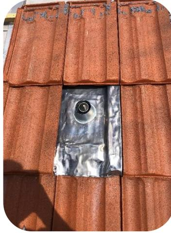
**H. PLACER LA CLOCHE DE RECOUVREMENT SUR LA TIGE FILETÉE DU PLOT SUPPORT**
