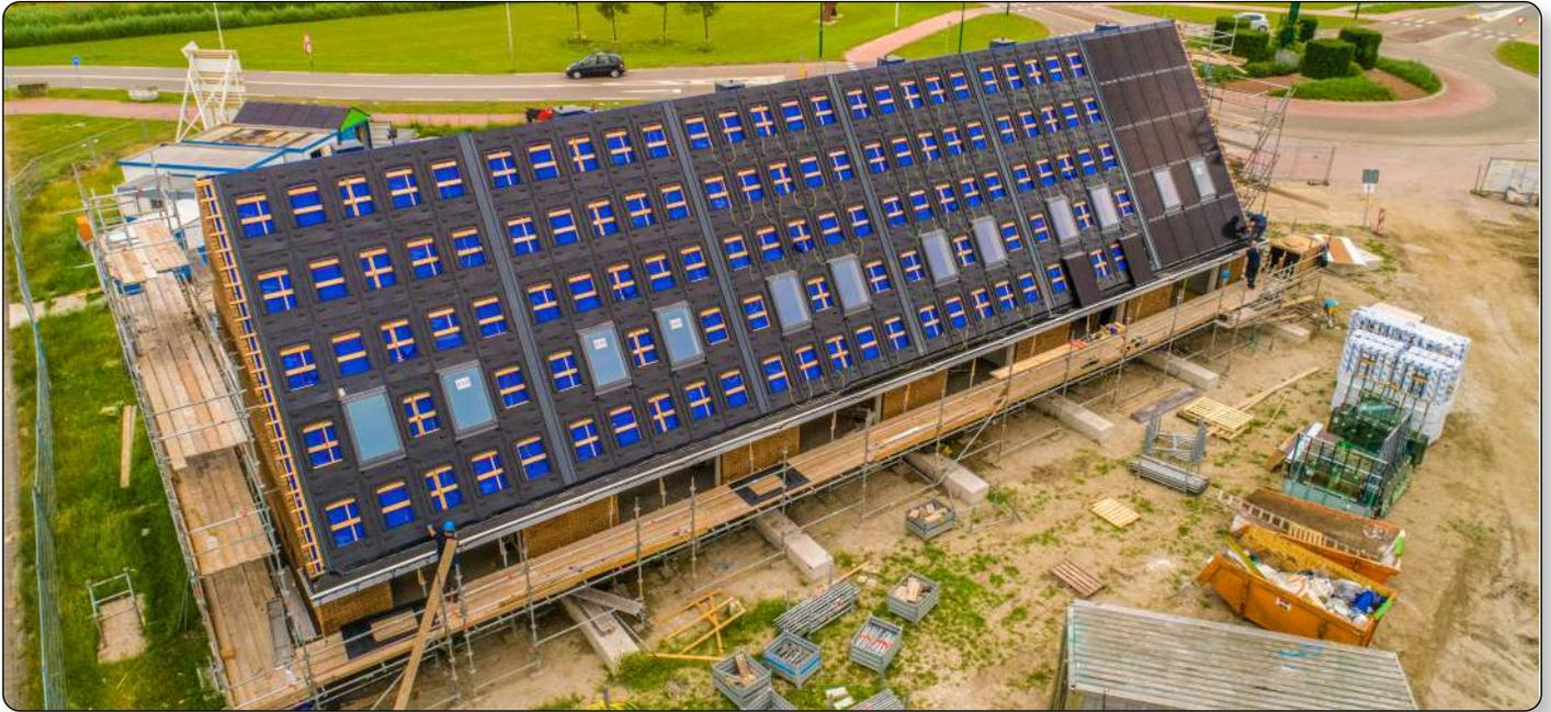
For more than 10 years, **GSE Intégration** has been developing an IN-ROOF mounting system that allows the construction of a solar roof with standard photovoltaic modules.
